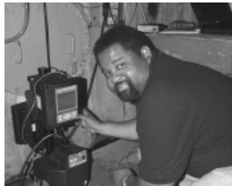
Russell Ford collecting data at a water treatment plant
